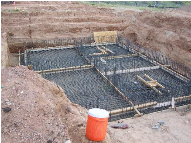
Rebar in floor of aerator and clarifier
